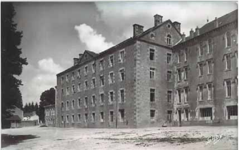
Figure 7: The back of the building
