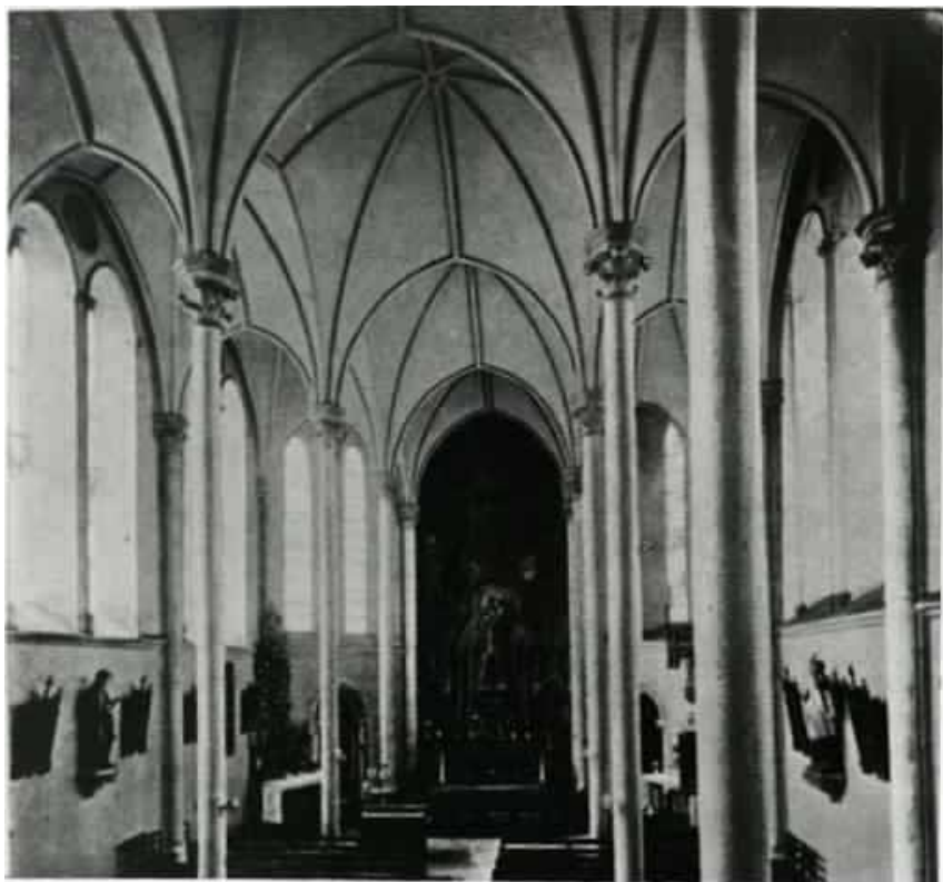
Figure 8: Interior of the church
