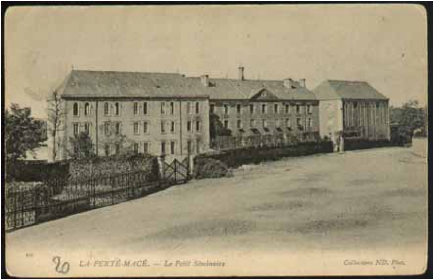
Figure 6: The front of the building
