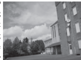
Figure 7, Asphalt court with far gate
