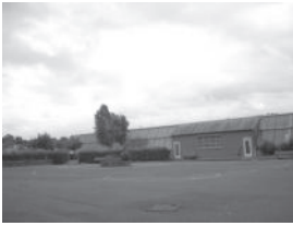
Figure 5, The greenhouse and shed
