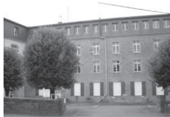
Figure 9, Middle building, front
